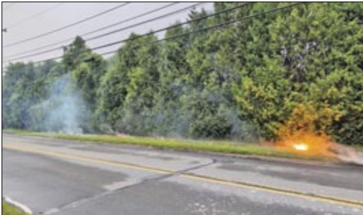
ABOVE: An electrical wire is on fire on the sidewalk on Sciticut Neck Road near Goulart Memorial Drive on 8/17/26. Photo by Scott Gobar. TOP: The ground is scorched where an electrical wire fell to the sidewalk. Photo by Beth David.
