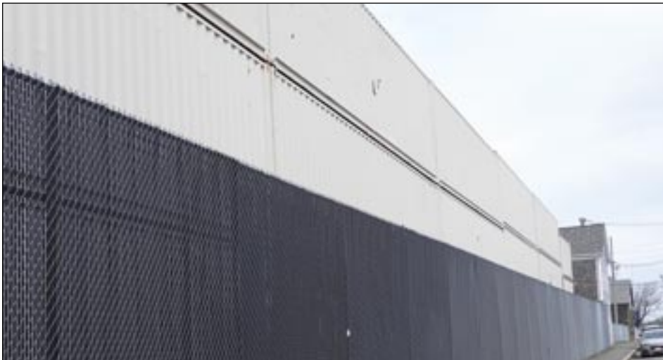
Shipping containers, such as these, will be allowed in more locations in Fairhaven "by-right" if the bylaw changes are passed at the Annual Town Meeting on 5/4/24. Photo by Wayne Hayward.
