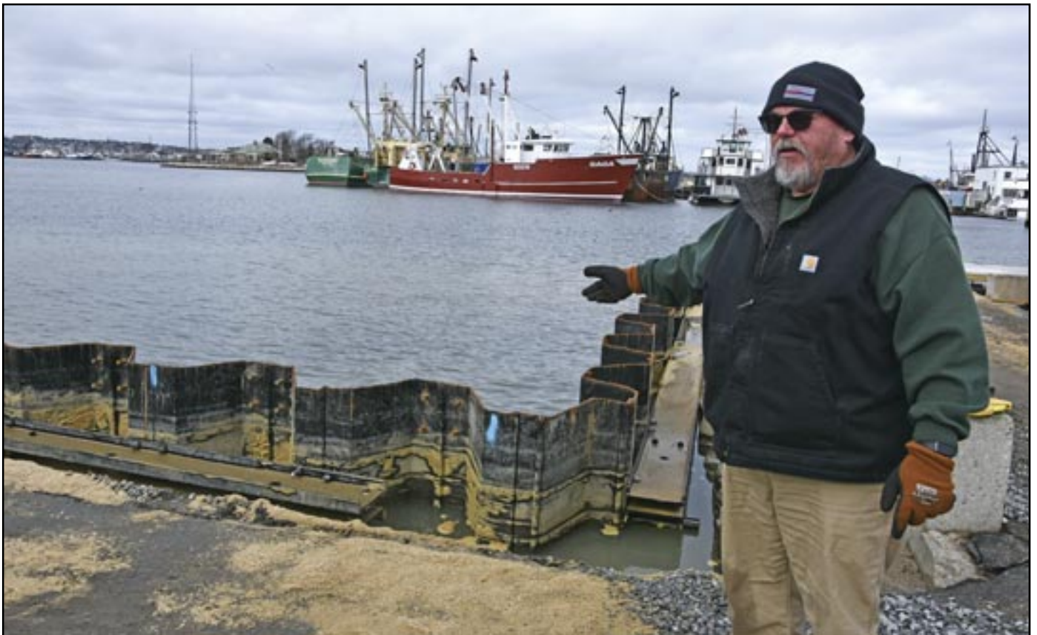
Fairhaven Harbormaster Tim Cox points out the "sheets" that form the frame of the wall at Union Wharf in Fairhaven, which are 50 feet long, with most of that length driven into the bottom. The i-beam holds the sheets together. Next will come concrete. The nearly $8 million project should be just about finished in April. See page 12. Photo by Beth David.
