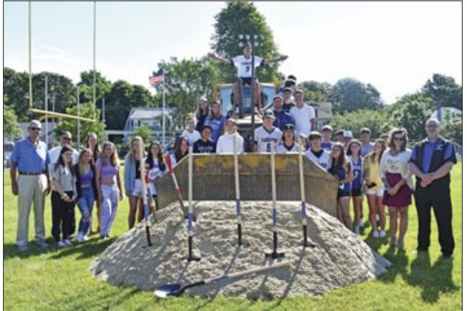
Fairhaven school officials, town officials, athletes, and others instrumental in getting the new Fairhaven High School turf field approved, attend the ceremonial groundbreaking on June 11, 2021. Submitted photo.
