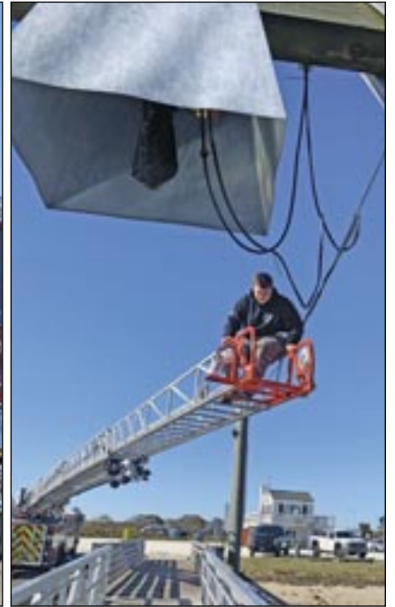
The bag that holds the winch chin for the gangway at Hoppy's Landing came loose in the last storm. When winds reach 50 miles per hour, the gangway is raised to protect it from being damaged. To re-attach the bag, the Fairhaven Fire Department helped out with Ladder 1, allowing Shellfish Warden/Deputy Todd Cox to reach the winch. Mr. Cox had to clean out a bird's nest, too, before re-attaching the bag with that holds the chain. LEFT & MIDDLE: Shellfish Warden/Deputy Todd Cox gets a lift from Fairhaven's Ladder 1 to re-attach the bag that stores the chain that holds the gangway at Hoppy's Landing on Saturday, 11/2/19. RIGHT: The bag, which is in the foreground, inside the winch hood, also had a bird's nest in it. Photo courtesy of Fairhaven Harbormaster's office.
